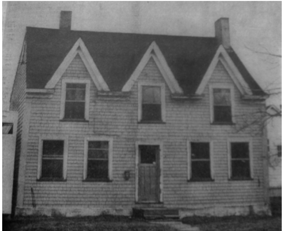
Cossit house before restoration. (Courtesy, Old Sydney Society)
