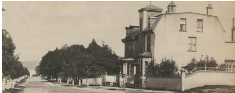
Uniacke-Sawyer house. (Courtesy of NSARM)
