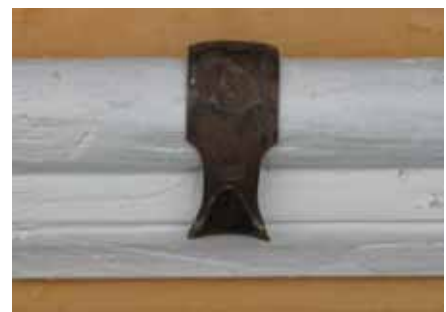
Face view showing hook and picture rail.
