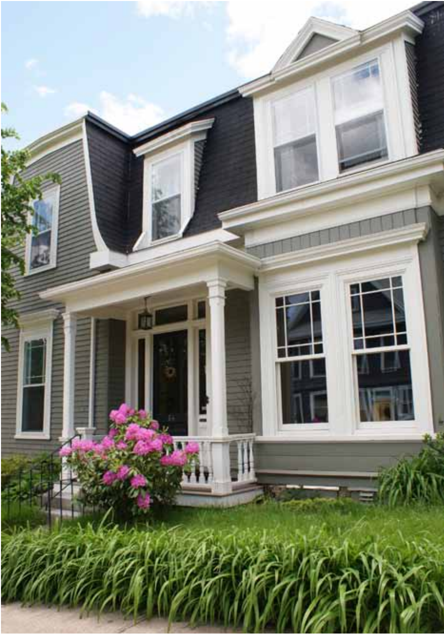
64 Queen Street. In The Story of Dartmouth , Dr. John Martin wrote about the aftermath of the Explosion that "patients were in the office and on the floors of the halls, dining room, living room and kitchen. Russell Urquhart, who was led by his brother from Hawthorne School... was placed on a fur coat [on the street] where Dr. Smith put 22 stitches in his mangled face... as fast as the boy's mother could thread the needles."
