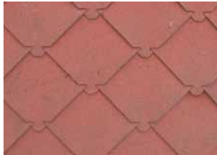
These vintage 12 inch diamond-lock asphalt shingles are actually square in shape but are installed in a diamond pattern. Location: Oxner's Barrel Factory, Chester Basin.
