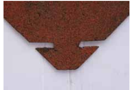
The bottoms of diamond-lock shingles were notched to lock into the adjacent shingles, providing maximum protection from wind.
