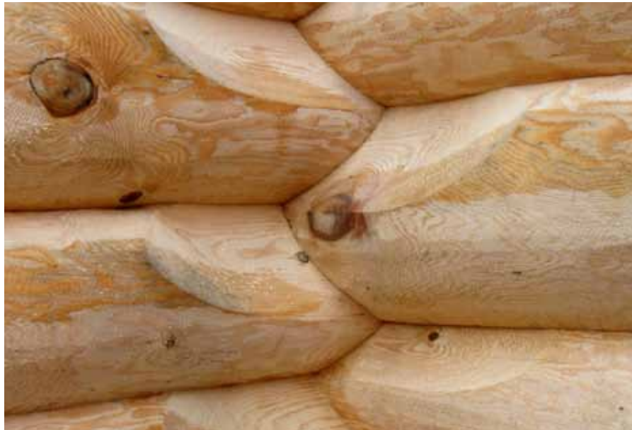
Photo 1: These saddle-notches were crafted by log-smiths Wade Hall and Roger Thomas of New Frontier Log Homes Ltd, New Ross.
