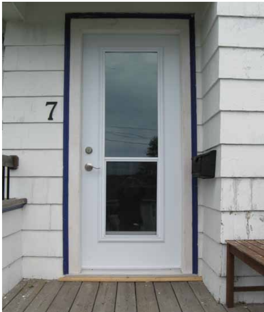
Photo 1A: Door and trim installed by author in Dartmouth, June 2011.
