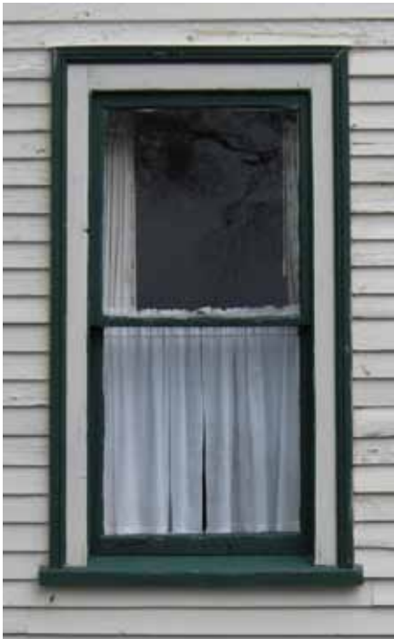
Photo 1B: Traditional trim with board and back-band sitting on sill extensions. Location: Robinson House, Chester.
