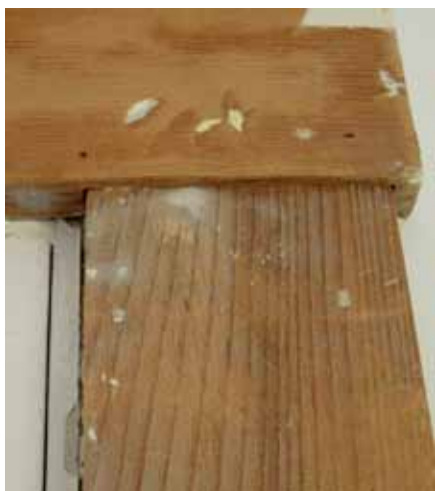
The side casing fits into a pocket on the underside of the head-trim. Notice the slight head-trim extension at right.
