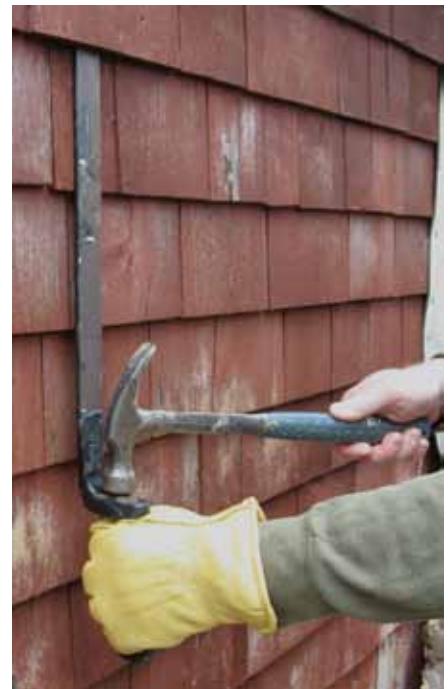
The shingle iron in action extracting nails hidden behind the shingles. Minimize hand injuries by wearing sturdy leather gloves.
