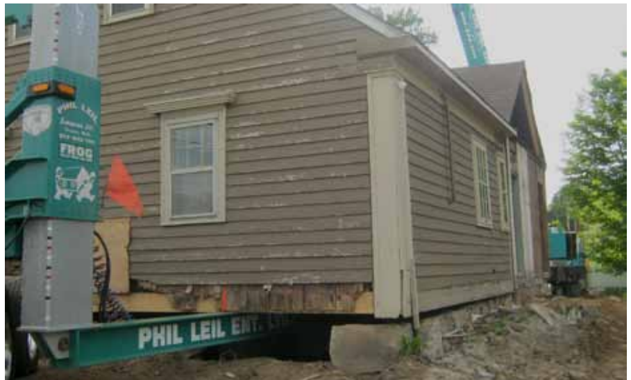
The house was very slowly raised for its move. (Courtesy of Su Rogers)
